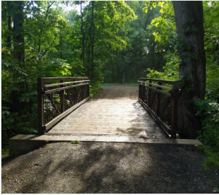
Mercer Meadows Bridge
